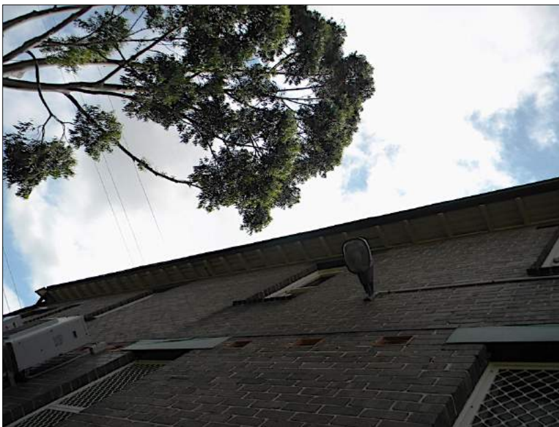
Figure 26: Detail of the timber lined eaves with exposed rafters.
