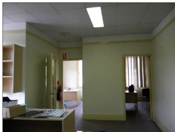
Figure 54: Original door with blocked in toplight and later door panel (Room 5).
