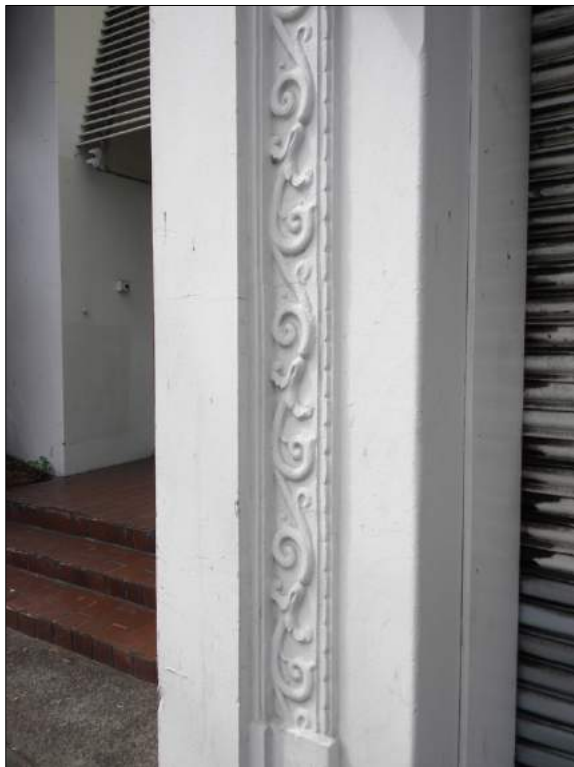
Figure 24: Detail of the decorative banding at ground floor level.
