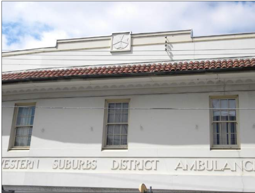
Figure 23: Detail of the first floor, showing the windows, shutter clips, lettering, decorative banding below the hood, cordova tiles to the hood and the Maltese Cross in the parapet.
