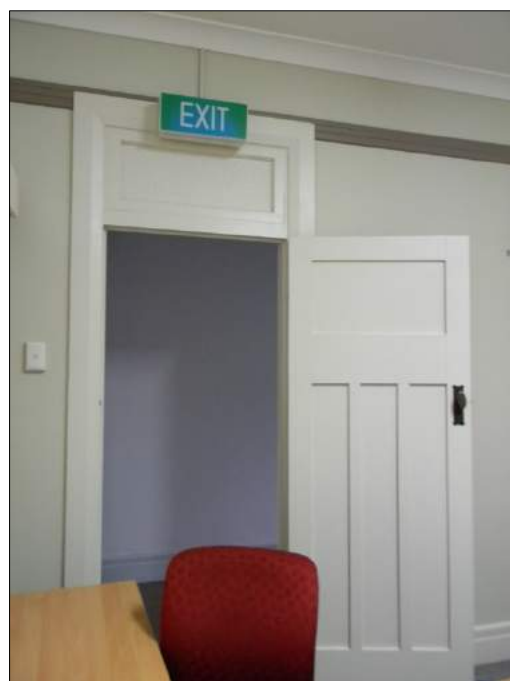
Figure 60: High waisted panel door with original hardware in Room G. The fanlight is blocked in.
