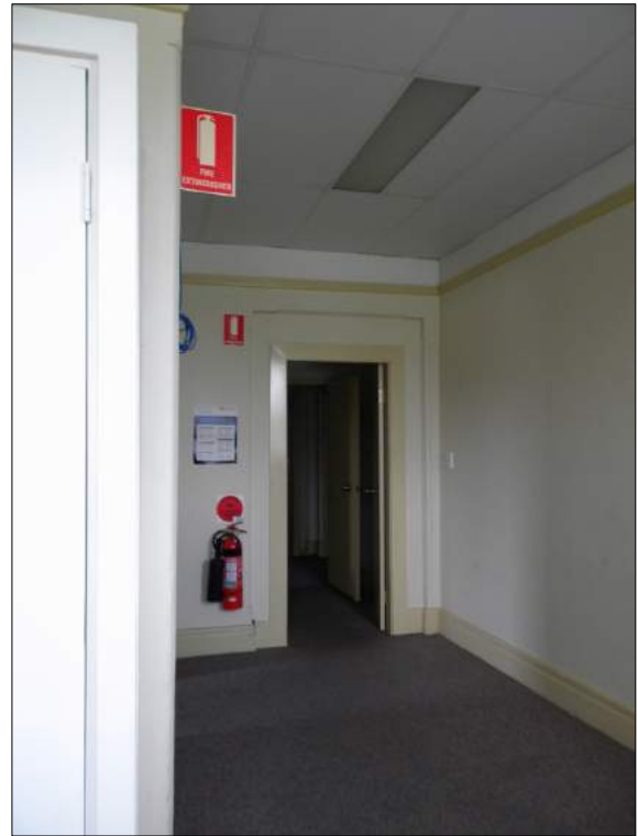
Figure 51: Door leading from Room 2 into Room 1. An earlier opening has been partially infilled and the door added.
