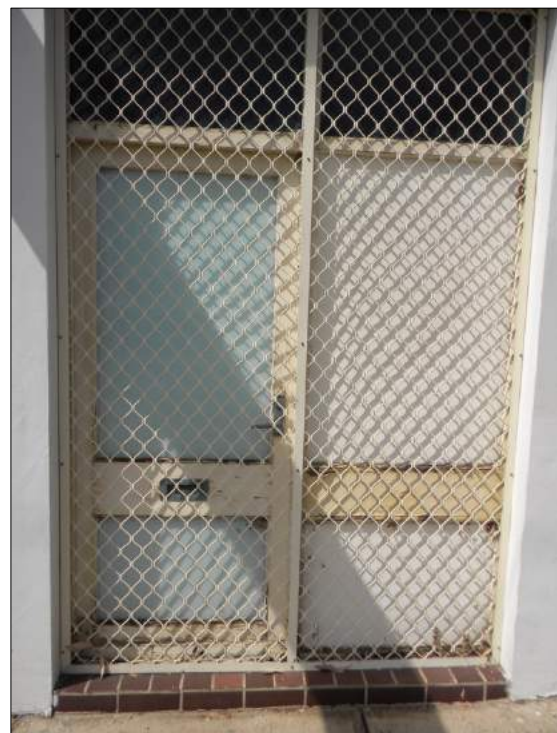
Figure 21: Detail of the main pedestrian access into the building. The floor is finished in no-original quarry tiles.
