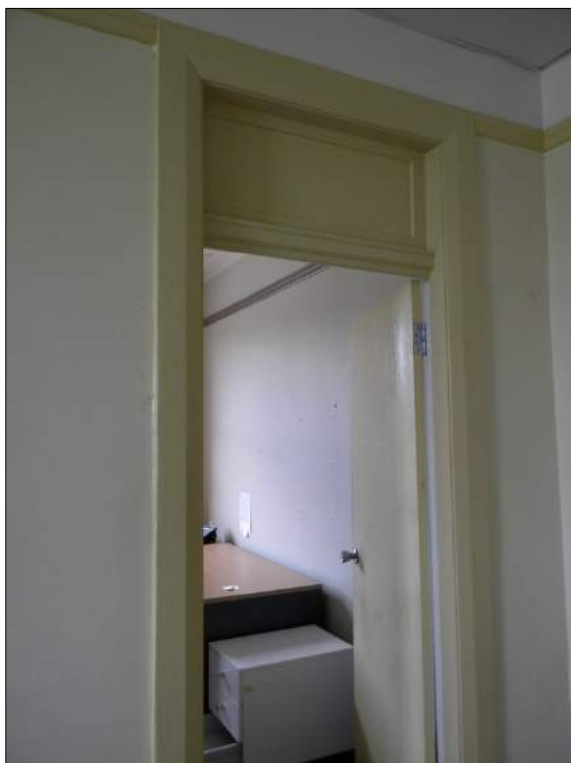
Figure 54: Original door with blocked in toplight and later door panel (Room 5).
